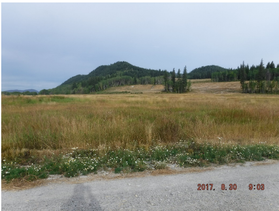
Photo II-2 Tailings Dam – East Leg, looking west at the covered tailings surface.
