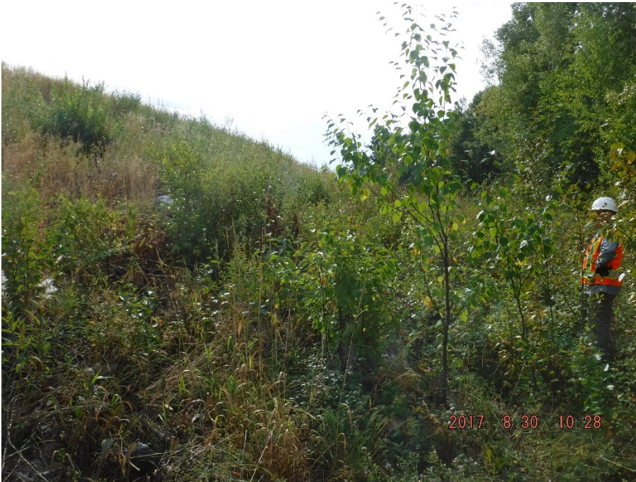
Photo II-17 Tailings Dam – West Leg, looking north along toe.
