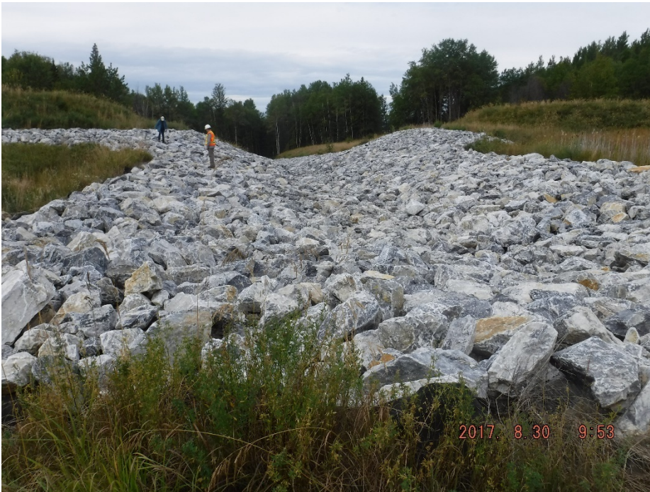
Photo II-19 Closure Spillway – Looking downstream from inlet area.
