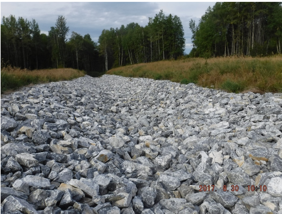
Photo II-22 Closure Spillway, looking downstream.
