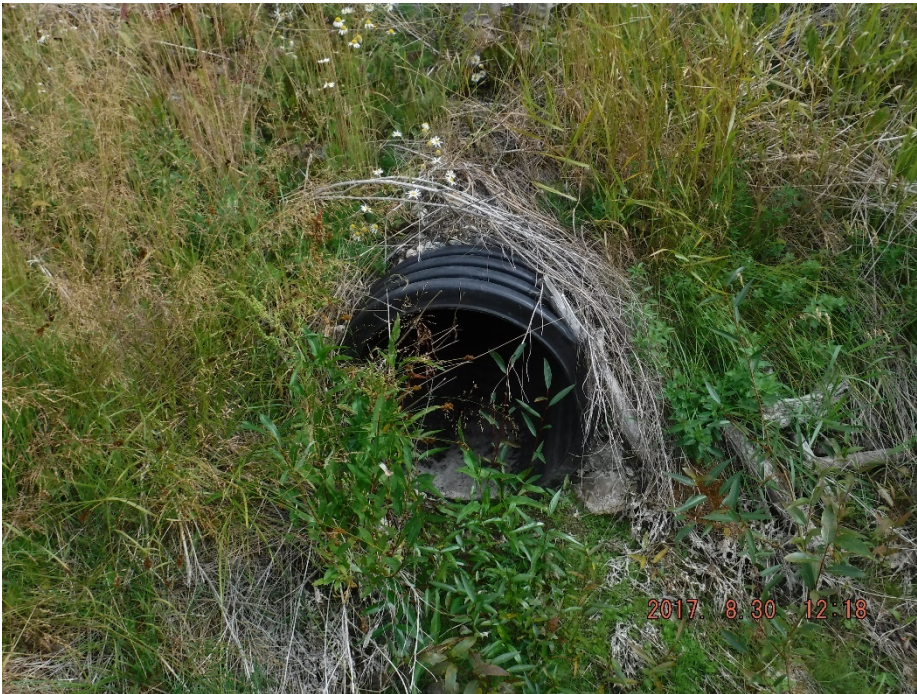
Photo II-29 Spillway Downstream Channel, outlet of culvert beneath road to caretaker's house.
