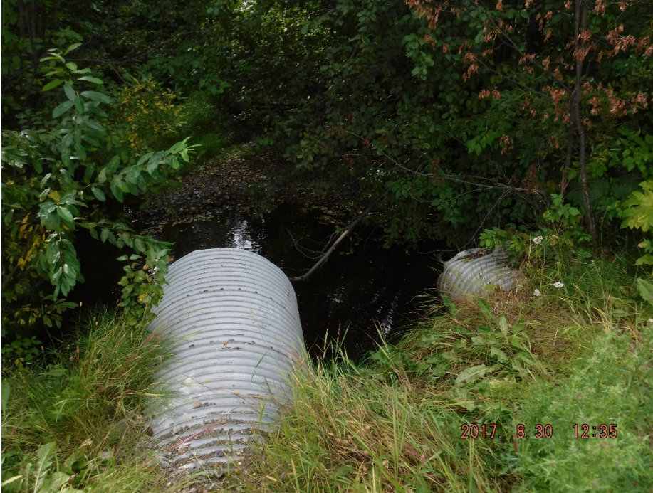
Photo II-49 Outlets of Ed Creek culverts under Pinchi lake Road.
