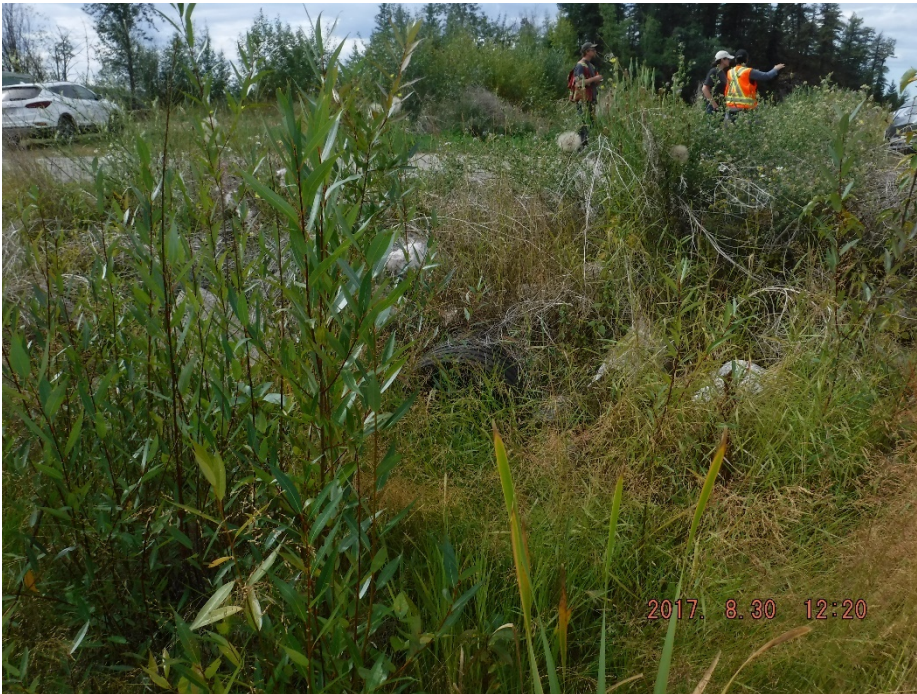
Photo II-27 Spillway Downstream Channel – inlet to culvert beneath road to caretaker’s house.
