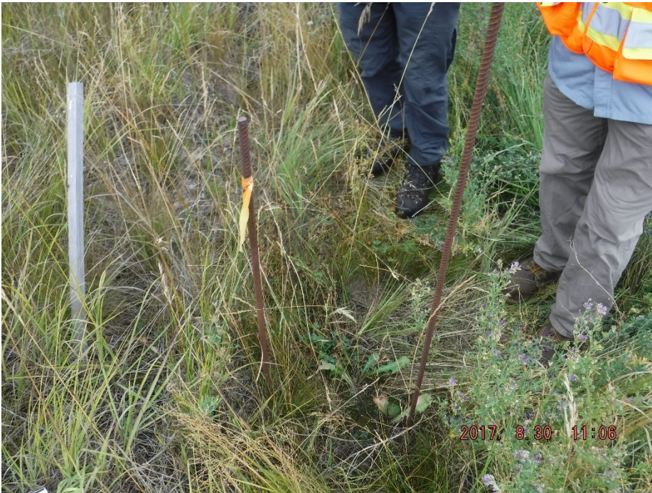
Photo II-31 Borrow Area A – tension crack monitoring rod location 403.
