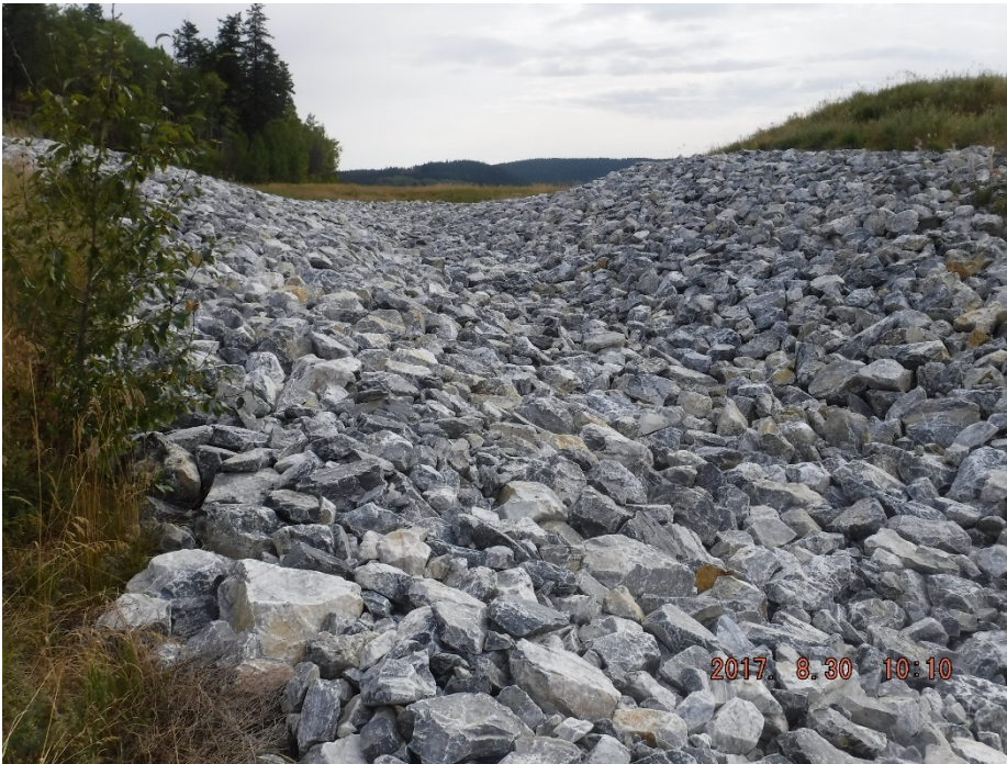
Photo II-21 Closure Spillway, looking upstream from dam toe area.
