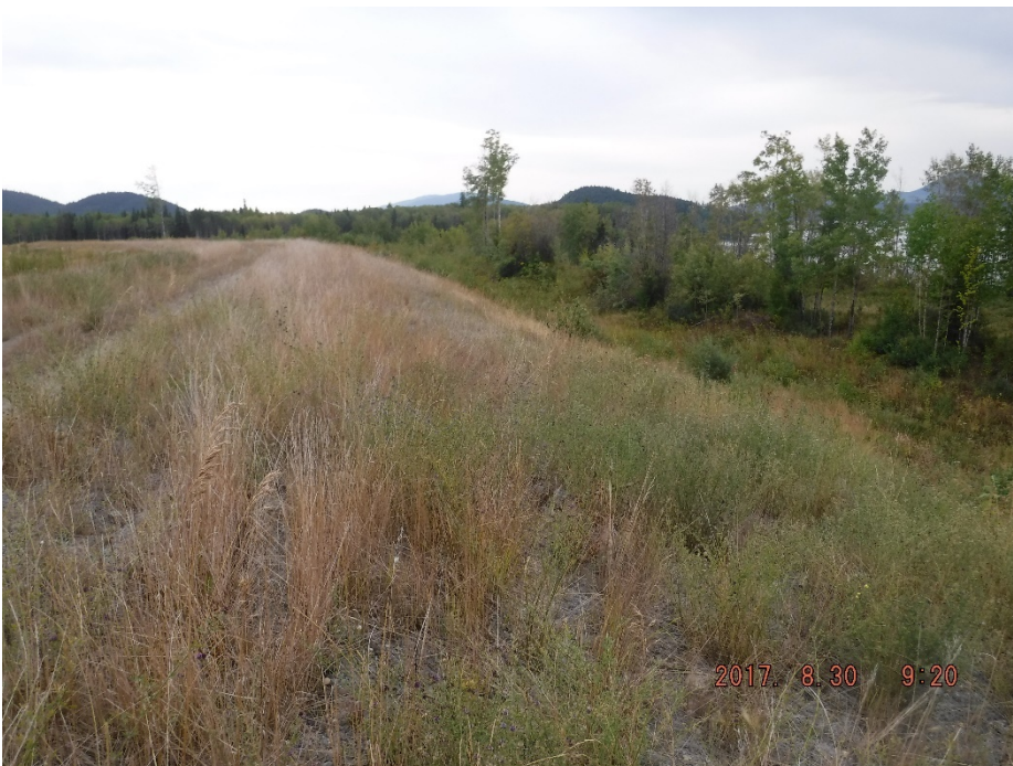
Photo II-8 Tailings Dam – Southwest Leg, looking southeast along downstream slope.
