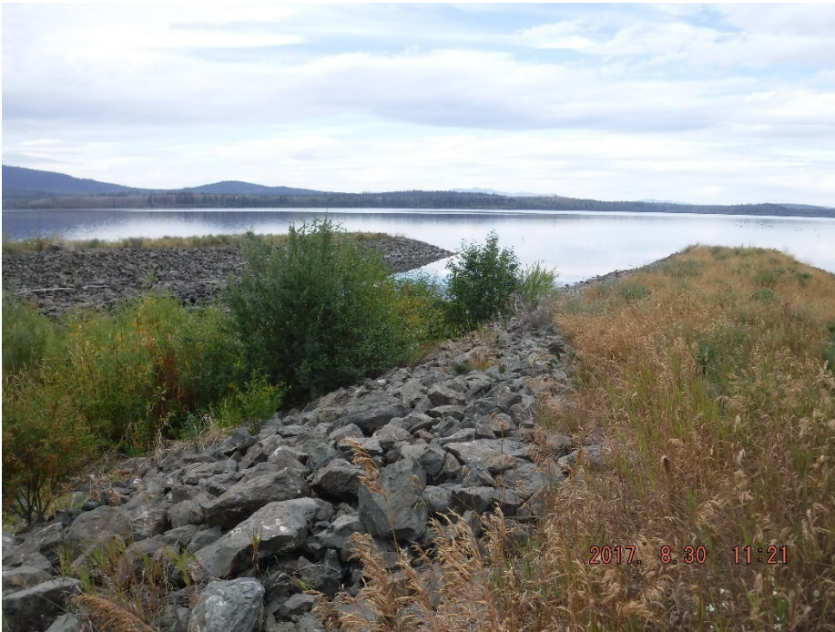
Photo II-37 Ed Creek Diversion Channel, outlet at Pinchi Lake.
