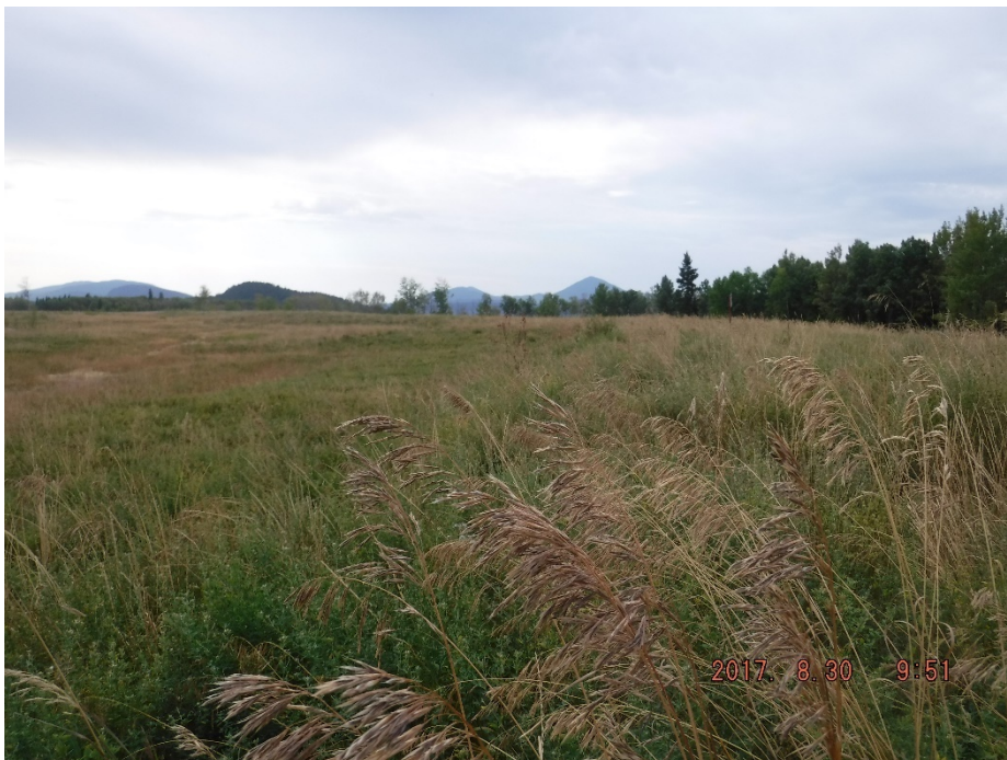
Photo II-16 Tailings Dam – West Leg, looking south along dam crest.
