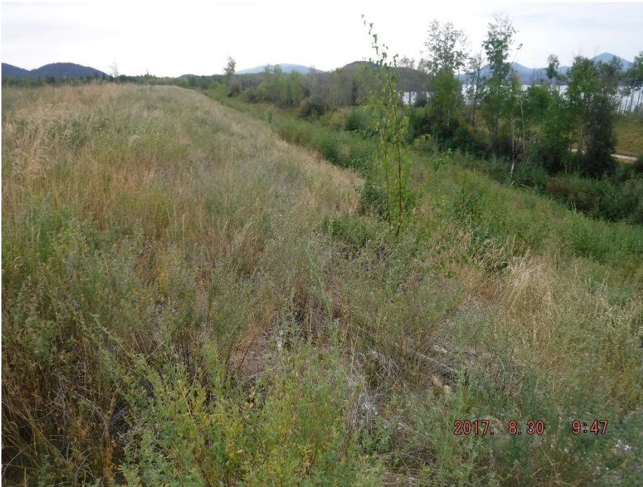
Photo II-11 Tailings Dam – Southwest Leg, looking southeast along downstream slope.
