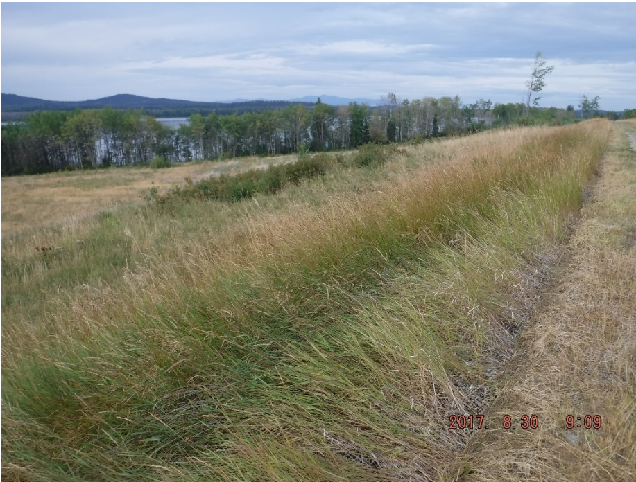
Photo II-5 Tailings Dam – South Leg, looking west along downstream slope.
