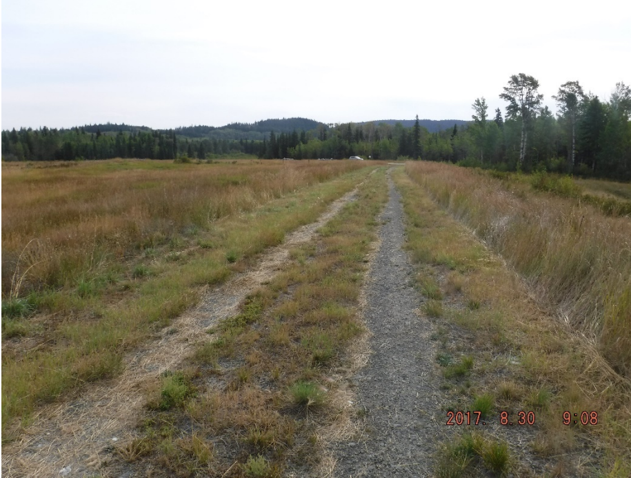
Photo II-3 Tailings Dam – South Leg, looking east from mid-point towards Ed Creek.
