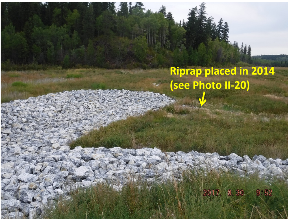
Photo II-18 Closure Spillway, inlet apron.
