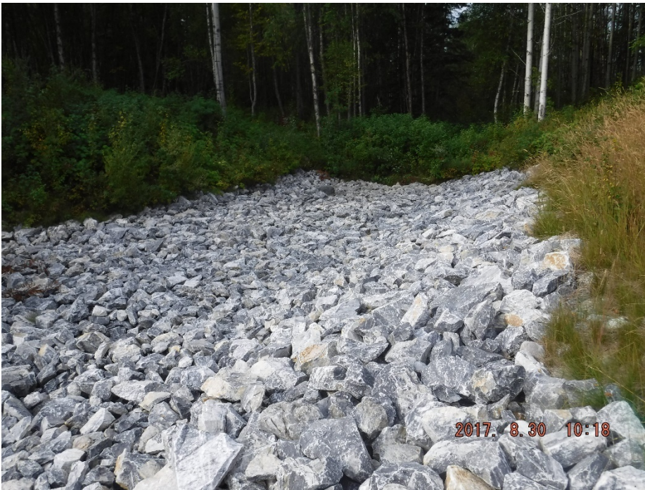
Photo II-25 Closure Spillway – looking downstream towards end of riprap-lined portion of channel.
