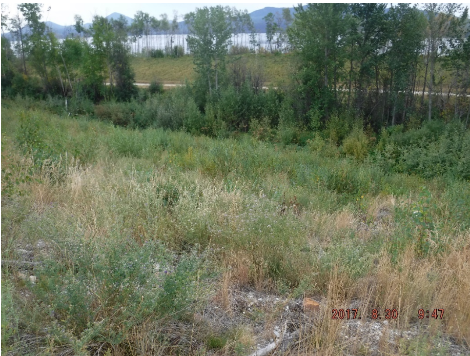
Photo II-12 Tailings Dam – Southwest Leg, looking downslope towards the toe.
