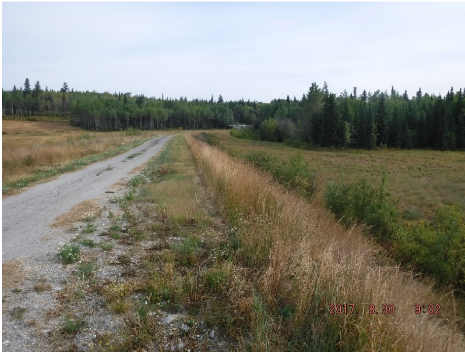
Photo II-1 Tailings Dam – East Leg, looking north towards the mine gate.
