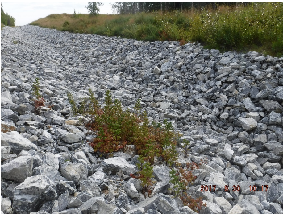
Photo II-24 Closure Spillway – looking upstream from near downstream end of channel. Some minor regrowth of vegetation has occurred in this area.
